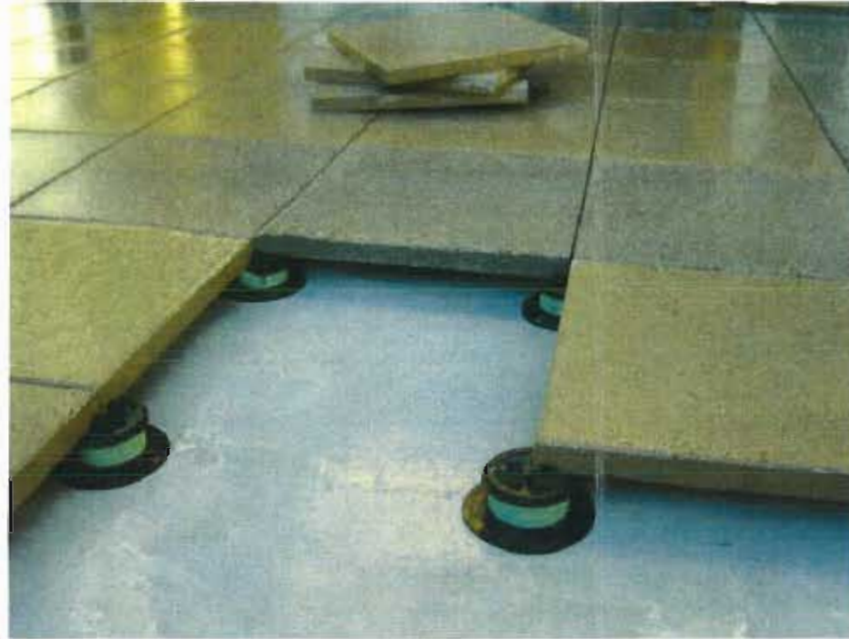
PRECAST CONCRETE PAVERS ON PEDESTAL
