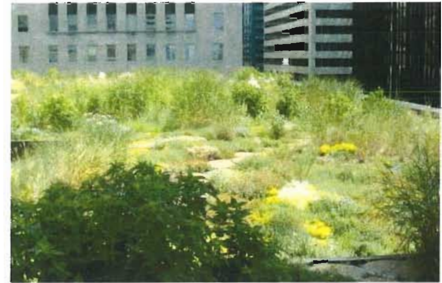
INTENSIVE GREEN ROOF PLANTINGS
