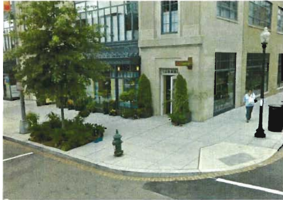
SCORED CONCRETE SIDEWALK
